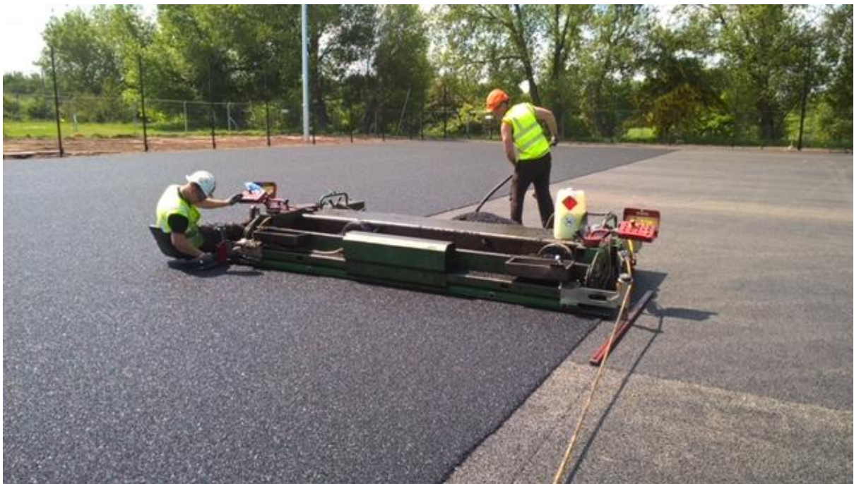
Picture: Shock pad layer being installed to England Hockey specification
