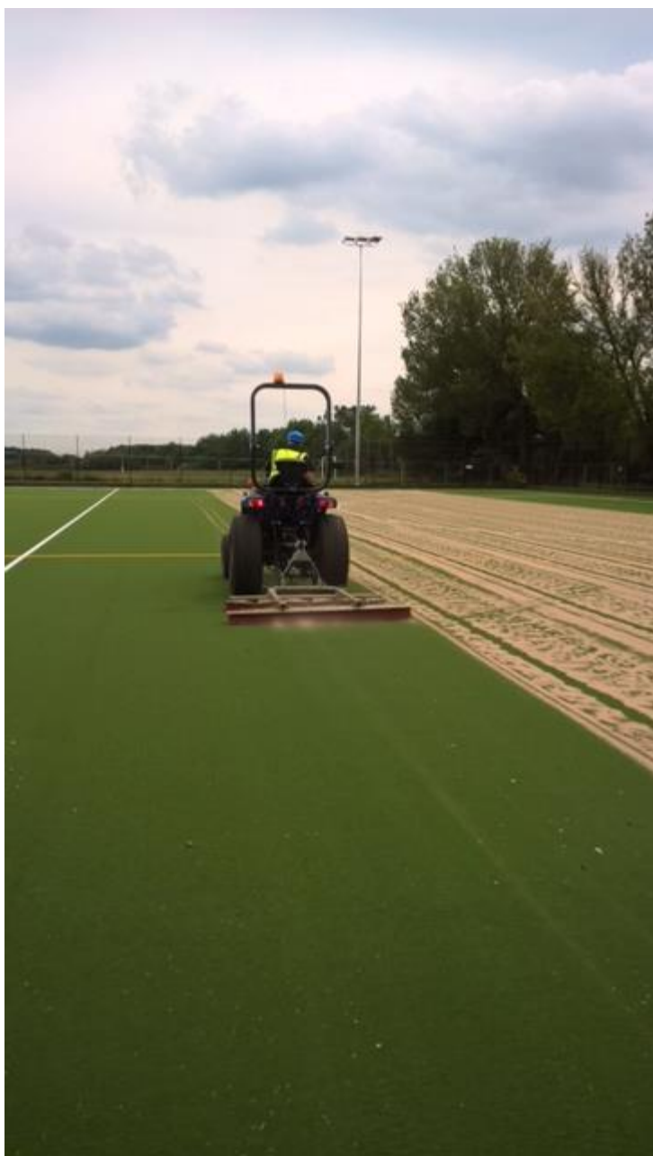
Picture: sand dressing the new pitch
