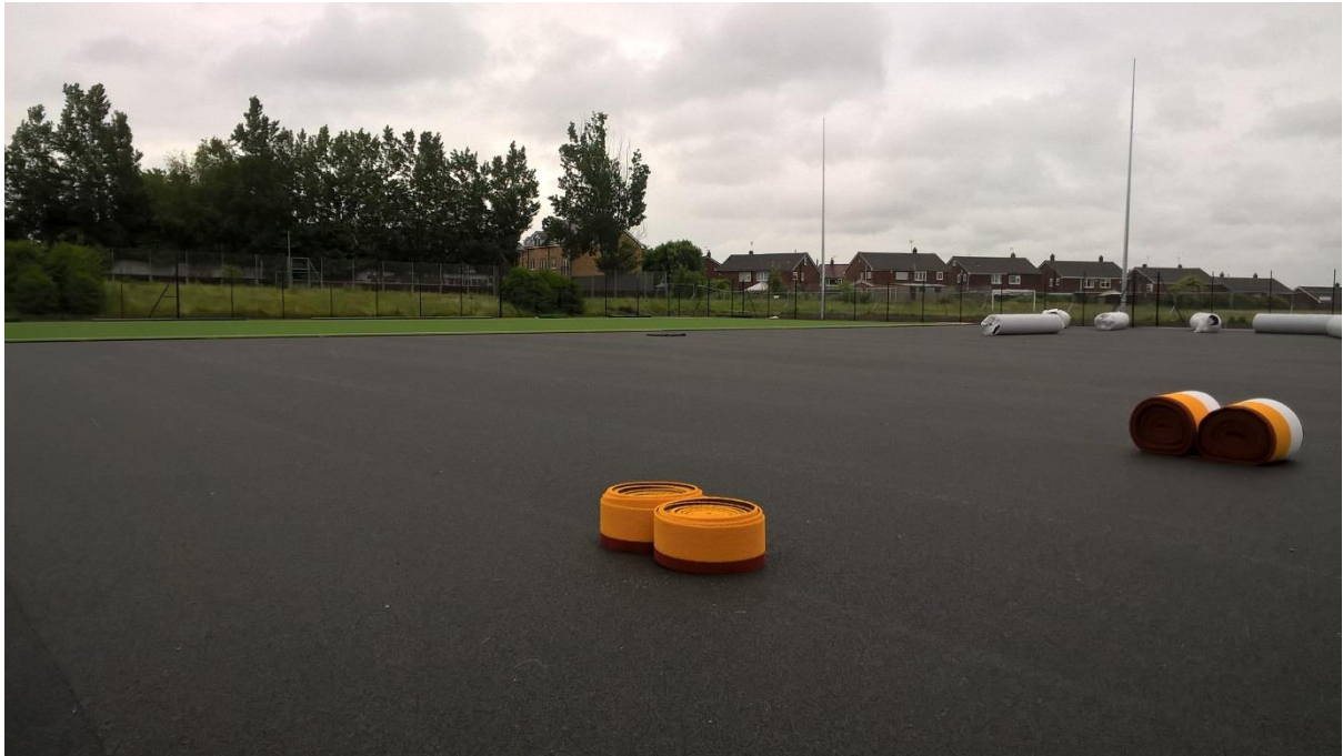
Picture: Shock pad layer being installed and new surface delivered
