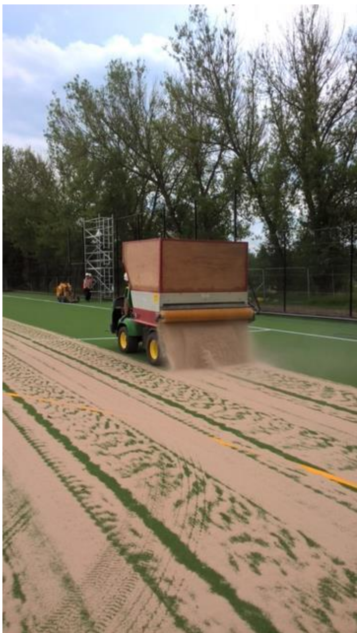
Picture: sand dressing the new pitch
